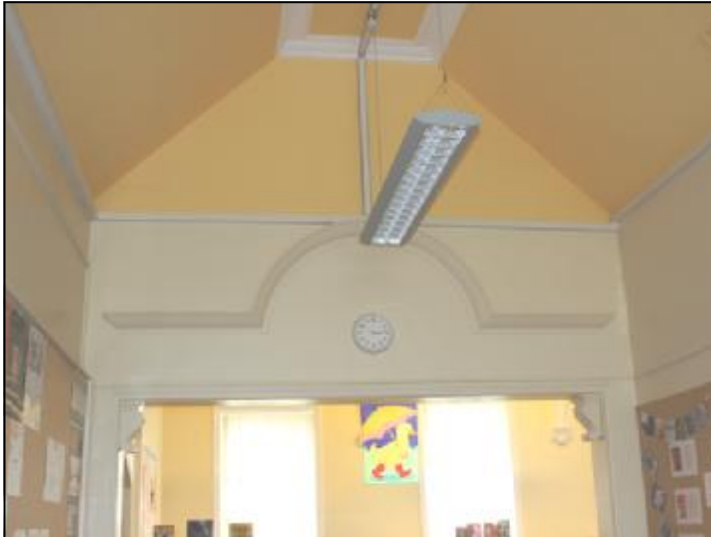
Plaster detail over room partition from room forty-seven to room fifty-one.
