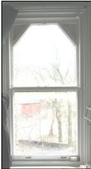
Window shape reflects similar shape elsewhere in the building
