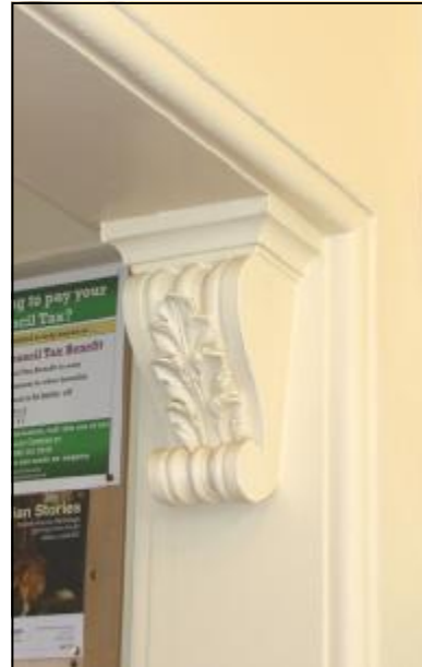
Corbel to room divider seen on left
